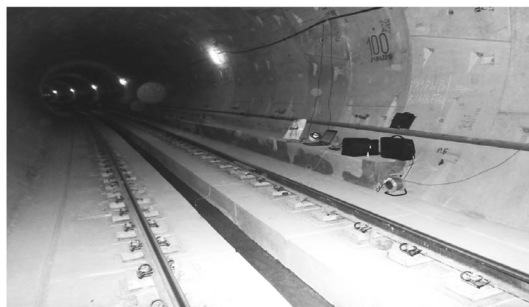
Figure 1. Appearance of the railway track and tunnel lining
